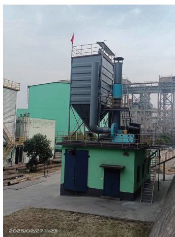
Belt corridor transfer station dust collector
